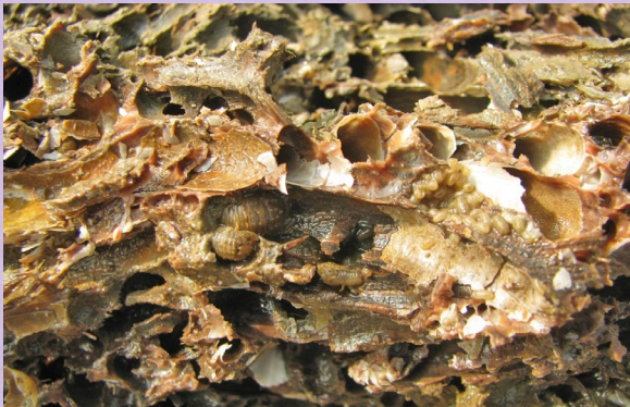
Attack of wood boring Isopod
